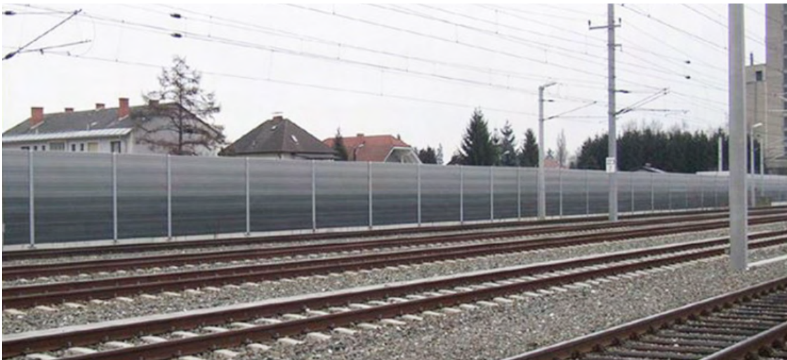
Figure 31b: aluminium cassettes have a modular design.
